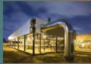
Advanced Oxidation Process (AOP) - Peroxide and UV
